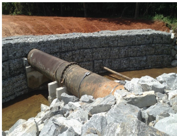
After Creek Bank Stabilization and Pier Rehabilitation
