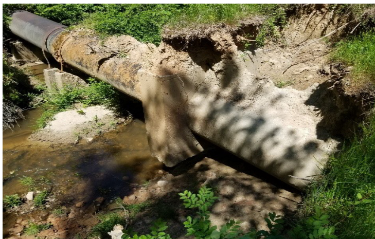
Before Creek Bank Stabilization and Pier Rehabilitation
