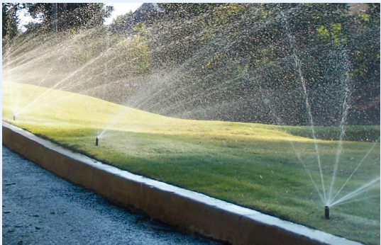
Sprinkler heads are only directed towards grass so that the pavement is not being watered.
