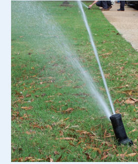
Improperly functioning rotor sprinkler head
