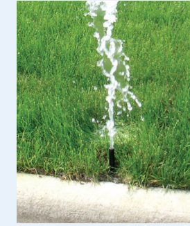
Improperly functioning rotor sprinkler head
