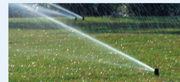
Properly functioning rotor sprinkler head
